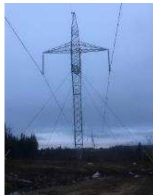
**FIGURE 6** Suspension tower without electrode lines
