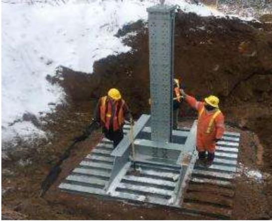
**FIGURE 11** Grillage foundation installed.
