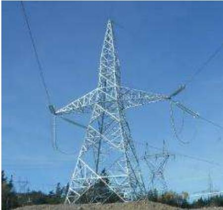
FIGURE 7 Tension tower without electrode lines
