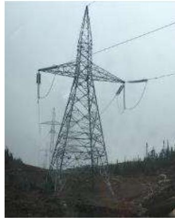
FIGURE 8 Tension tower without electrode lines
