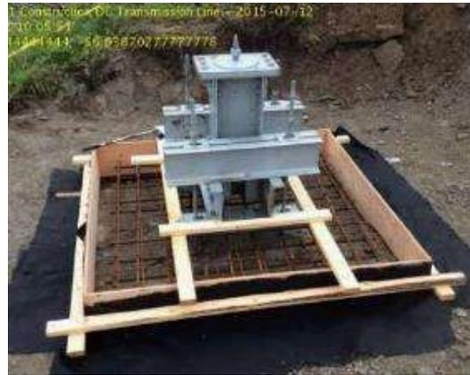
**FIGURE 14** Rock foundation, ready for concrete.
