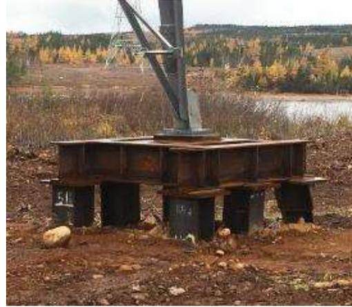
**FIGURE 12** Pile foundation.
